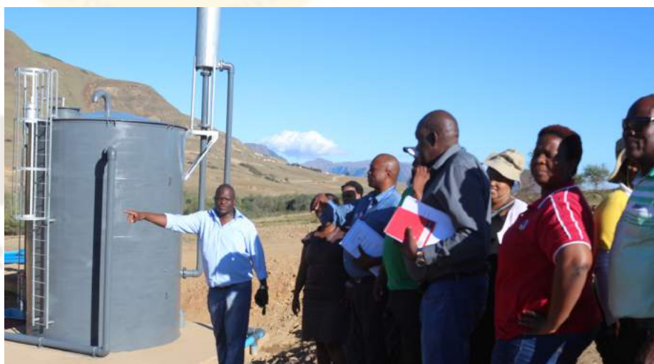
Above: MPAC delegation inspecting Ntibane/Mkhemane water scheme in Mount Frere
