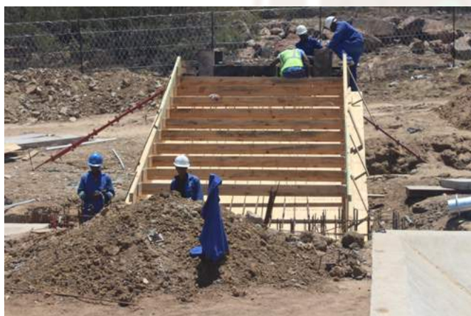
Above: Fobane water treatment works is still under construction in Matatiele
