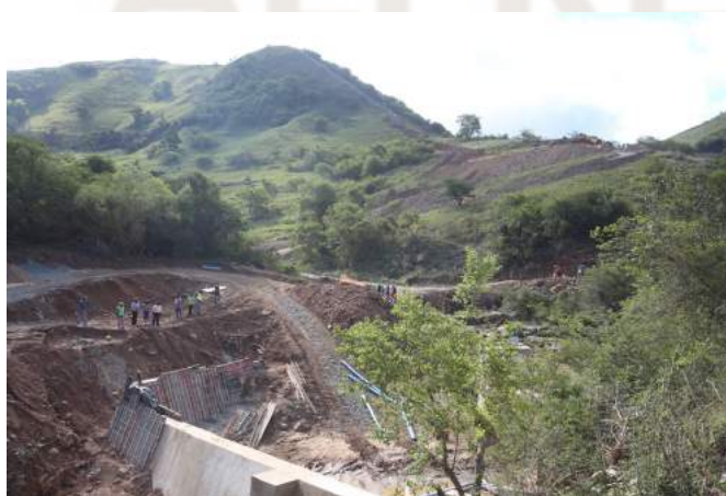
Above: construction of Bomvini/Nyokweni water scheme in progress
