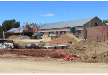
Above: Phase 3 construction at Khotsong TB Hospital in Matatiele.
