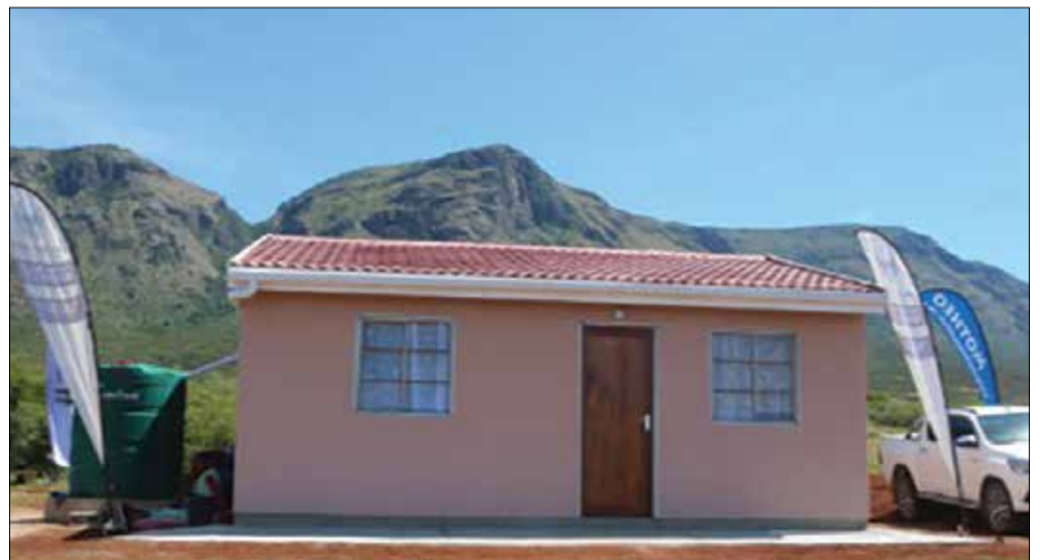
Above: A newly built permanent structure with furniture for Mrs Ncediswa Ndawule
